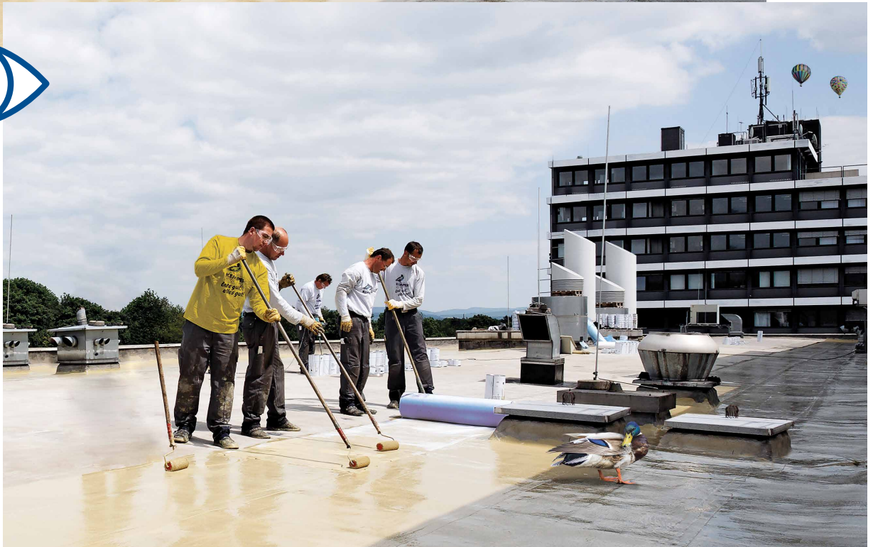
Application of KEMPEROL on the roof of the HNA printing centre Kassel, 2008.
