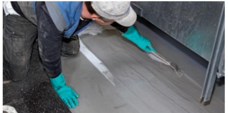
KEMPEROL® is liquid-applied waterproofing with fleece reinforcement.
