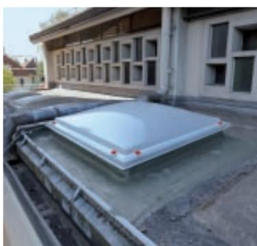
The first skylight dome coated with KEMPEROL® FALLSTOP was installed as a sample for final approval and waterproofed with KEMPEROL® 2K-PUR.
