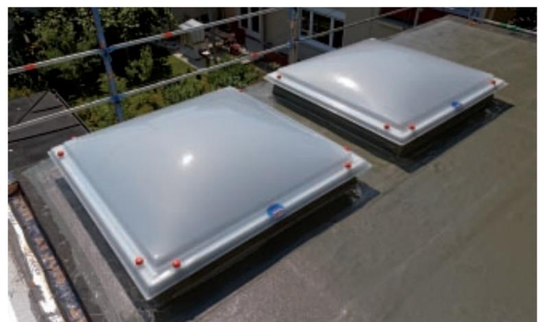
Fully installed skylight domes coated with KEMPEROL® FALLSTOP. The surface of the coated skylight domes has a slightly bluish shimmer.
