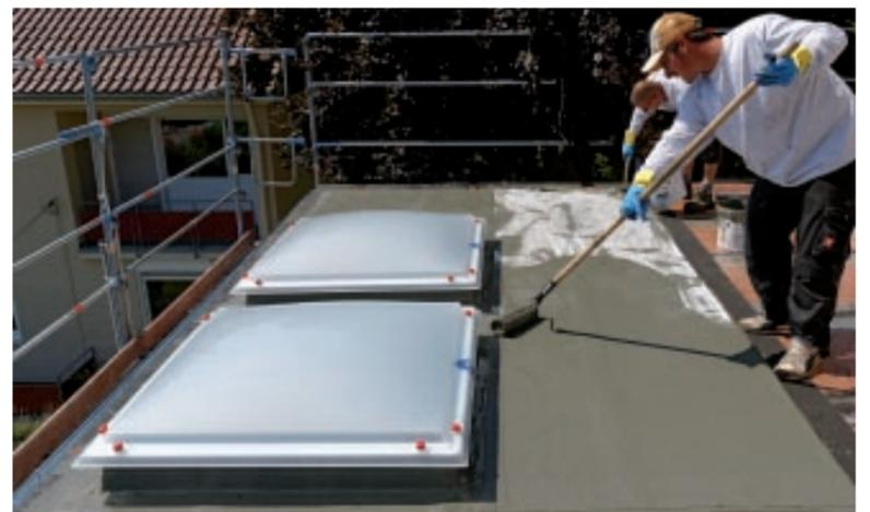
After installing the skylight domes, the roof was waterproofed with KEMPEROL® 2K-PUR.
