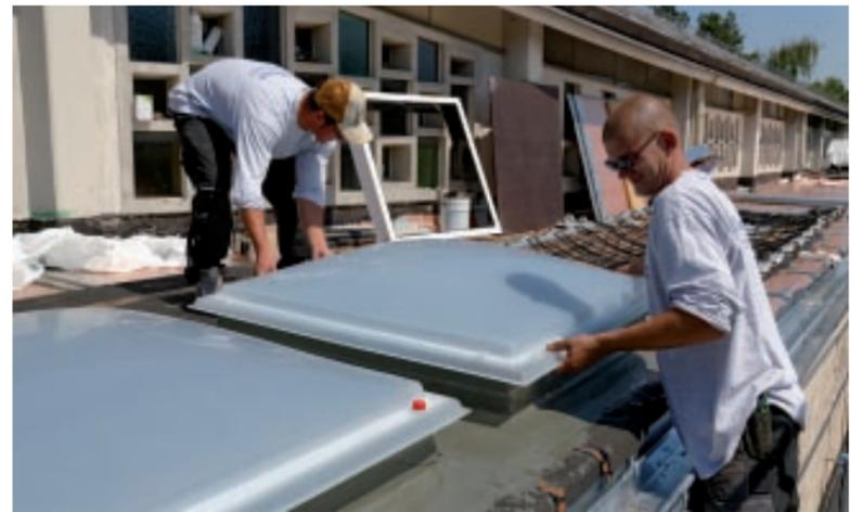
Finally, the dome coated with KEMPEROL® FALLSTOP is installed.
