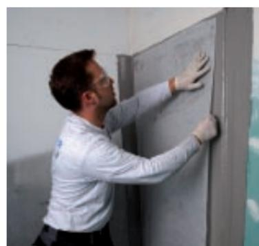
3 Reinforcement fleece covers all small cracks...
