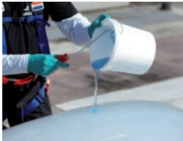
The ready-for-use KEMPEROL® FALLSTOP coating is then applied evenly and free of bubbles in four steps using a foam roller in a criss-cross fashion.
