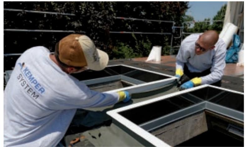
Waterproofing takes place in a confined space. The reinforcement fleece soaked in KEMPEROL® is applied directly to the sanded bitumen sheeting.
