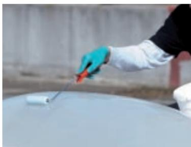
The surface is fully cured and fall-through protected after approx. seven days (at 23°C).
