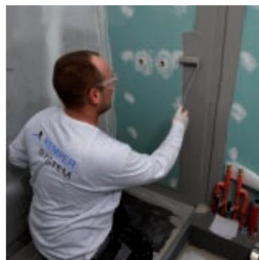
1 Easy handling: the liquid waterproofing system is applied with a roller.
