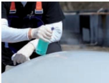
KEMPEROL® FALLSTOP can be applied quickly and easily. The surface must be cleaned thoroughly with KEMPERTEC® FALLSTOP Cleaner prior to application.
