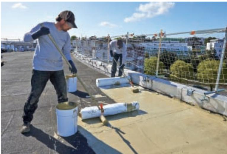
**The EHPAD\* in Nantes chooses KEMPEROL® 2K-PUR, the liquid-applied waterproofing solution for HQE\*\* conformity for the renovation of an 1100 m<sup>2</sup> flat roof on a sensitive residential development**
