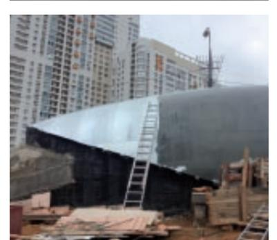
The bottom metal layer of the double-skinned metal structure was fully waterproofed using KEMPEROL®.
