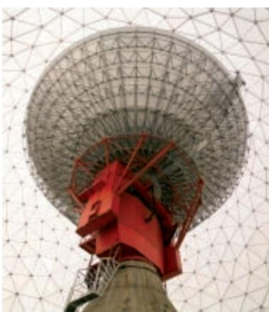
The horizontally and vertically adjustable parabolic reflector inside the dome measures 34 metres in diameter and weighs 240 tons.
