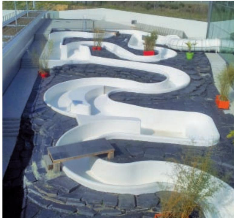
KEMPEROL® 2K-PUR is a solvent-free product, like the chosen coating, KEMPERDUR® Deko 2K, both being adapted to green buildings and sensitive environments, where the solvent vapours are not wished. The waterproofing has to be able to match all forms perfectly.
