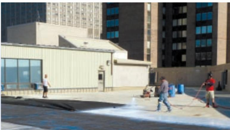
The KEMPEROL® 2K-PUR reinforced waterproofing membrane and the RUBBERWAY®-VersaCoat recreational surface were tested for compatibility. An acrylic adhesive is spray applied to the KEMPEROL® membrane to adhere the first of multiple layers of the sports surfacing.
