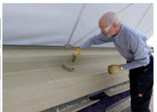
KEMPEROL® Waterproofing only came into contact with the special plastic fabric at the junction points, which were waterproofed separately.
